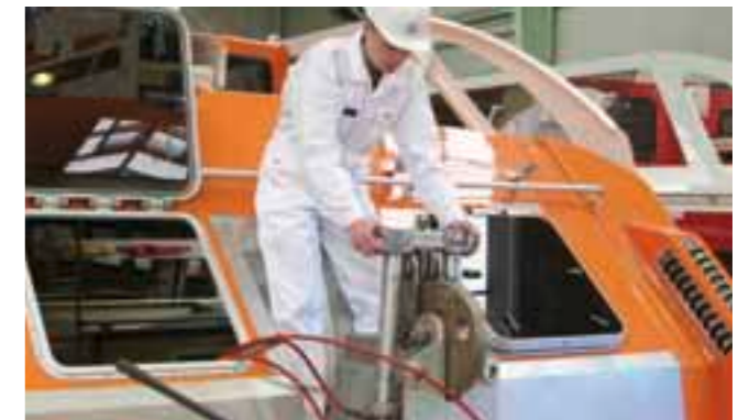
Overload test of release mechanism
