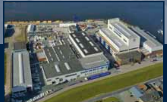
Fassmer Headquarters Germany | Berne
